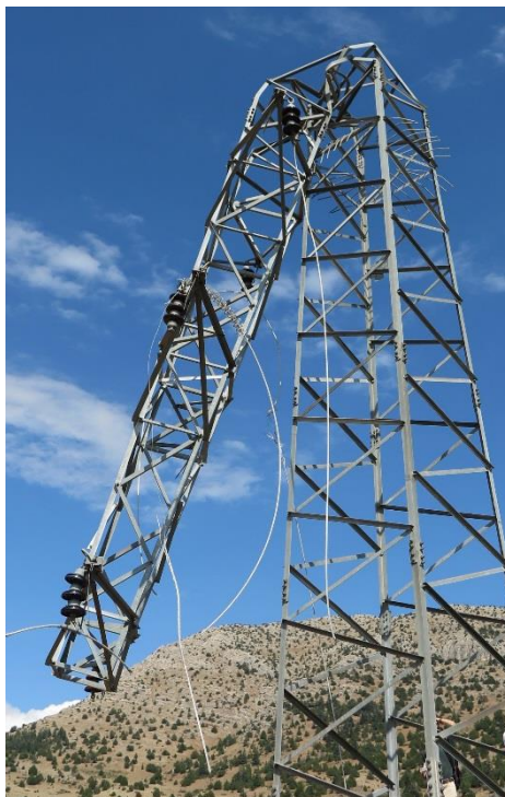
Figure B.2. No.107 tower (Buckling of leg members in tower body)
