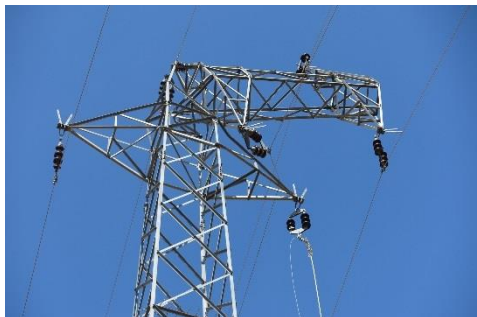
Figure B.4. No.116 tower (Torsional deformation of the tower cage between the middle and bottom crossarms)
