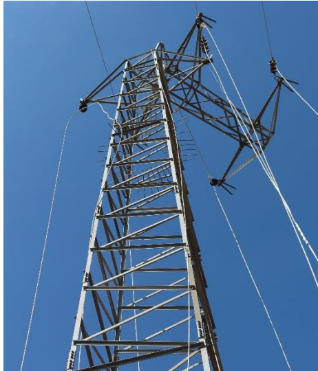
Figure B.1. No.106 tower (Torsional deformation of the tower cage between the middle and bottom crossarms)
