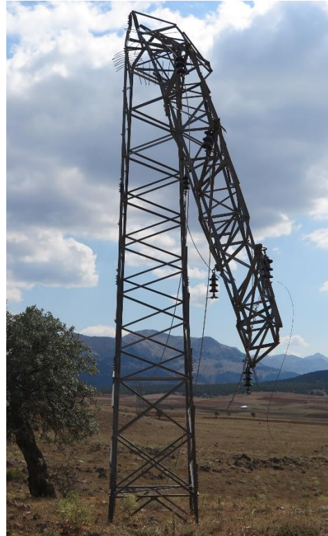
Figure B.3. No.108 tower (Buckling of leg members in tower body)
