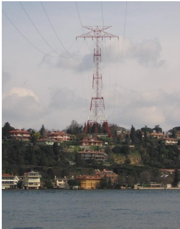
Figure 1.1. 154 kV Bosphorus crossing steel lattice transmission tower
