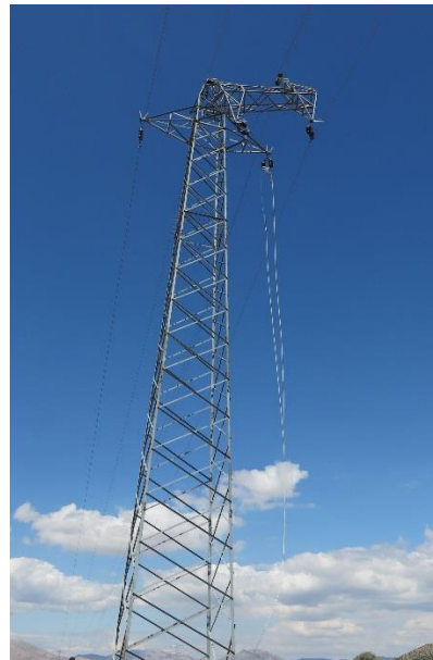
Figure B.4. No.116 tower (Torsional deformation of the tower cage between the middle and bottom crossarms)
