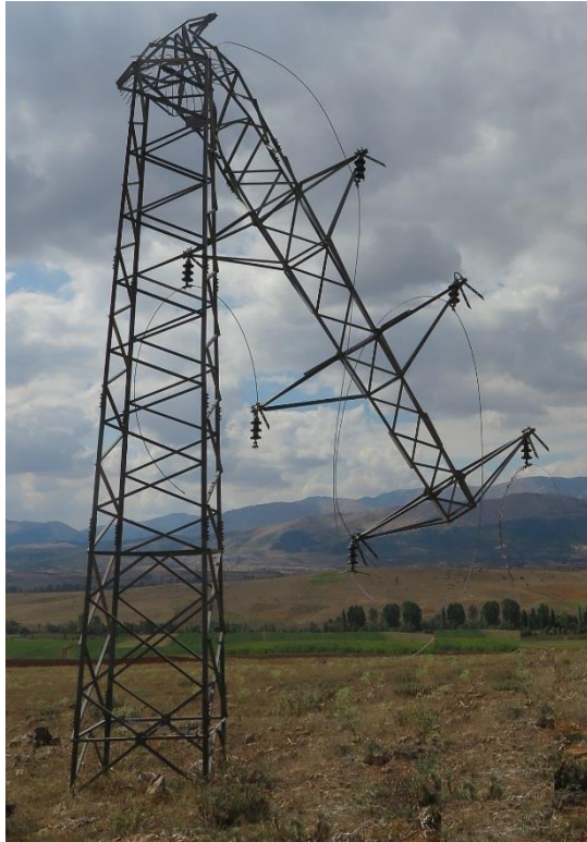
Figure B.3. No.108 tower (Buckling of leg members in tower body)
