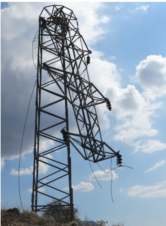
Figure B.2. No.107 tower (Buckling of leg members in tower body)
