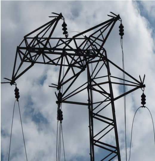
Figure B.1. No.106 tower (Torsional deformation of the tower cage between the middle and bottom crossarms)
